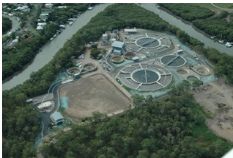
Sandgate Wastewater Treatment Plant
