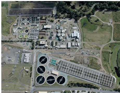
Oxley Creek Wastewater Treatment Plant
